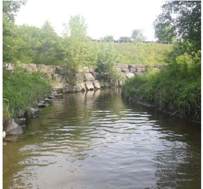
A highly altered section of Sawmill Creek where armour stone has been used to protect urban infrastructure at the top of the bank from the effects of stream erosion
