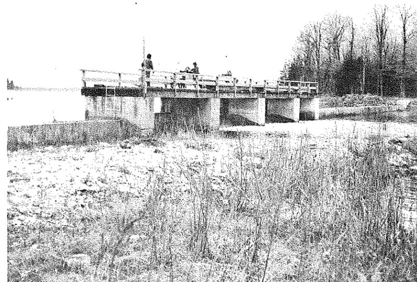
PHOTO 2    STOP LOG BAYS AT BEVERIDGE DAM
