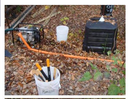
Pump to carry water from isolated work area up the slope and into a silt bag which filters the water and holds the sediment
