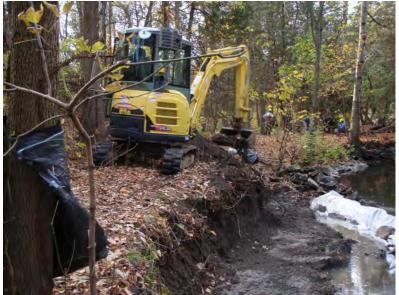
Machinery digging out base of bank to install first layer
