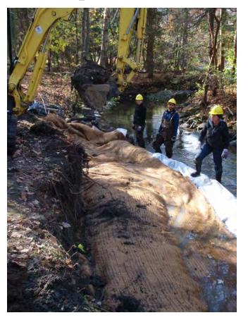
After willows and dogwoods are laid, the wrapping materials are laid down and filled with soil
