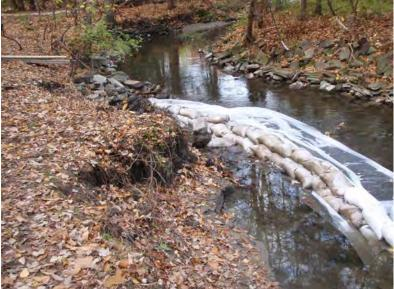
Isolated work site to prevent sediment from flowing into the stream
