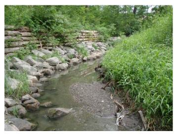
Photo 10. Existing rip rap and wooden retaining wall installed by as part of the City of Ottawa Erosion Control Works on Taylor Creek.
