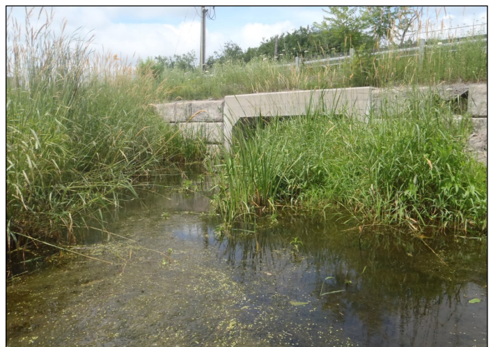
Roadway infrastructure on Corkstown Road along Stillwater Creek
