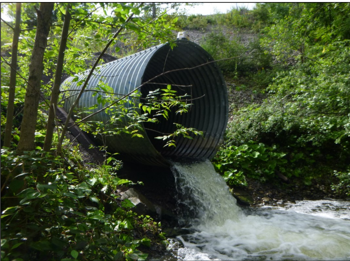
Perched culverts create fish migratory obstructions and loss of aquatic habitat and seasonal grounds for many fish species
