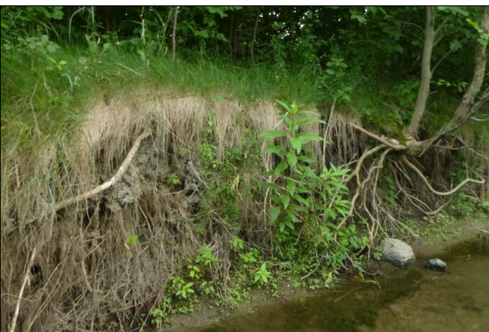
Bank erosion along Stillwater Creek upstream of HWY 417
