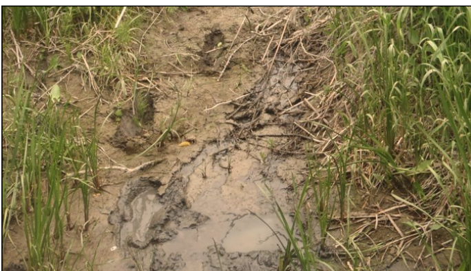
Substantial sediment deposition observed in a headwater drainage feature on Mud Creek.
