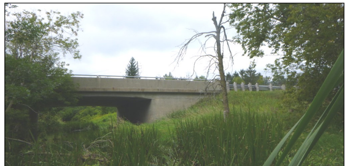
Roadway infrastructure on Prince of Wales Drive along Mud Creek.
