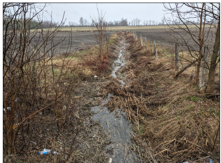
An example of historical channel straightening on a headwater drainage feature near Malakoff Road.
