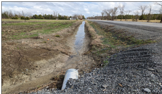
Headwater feature with no in-stream vegetation on Bankfield Road.
