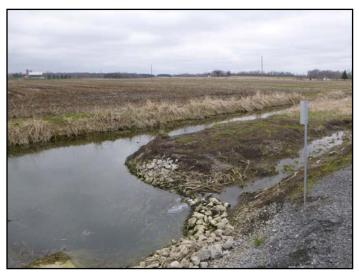
An example of mixed modifications on a headwater drainage feature: dredging and channel hardening with rip rap on Fourth Line Road
