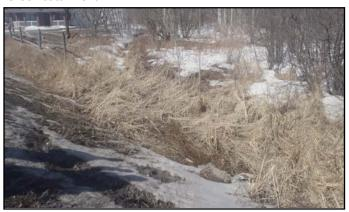
Substantial sediment deposition observed on Navan Road
