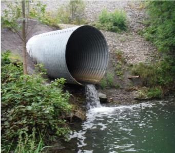
A perched culvert observed along a tributary of Stillwater Creek
