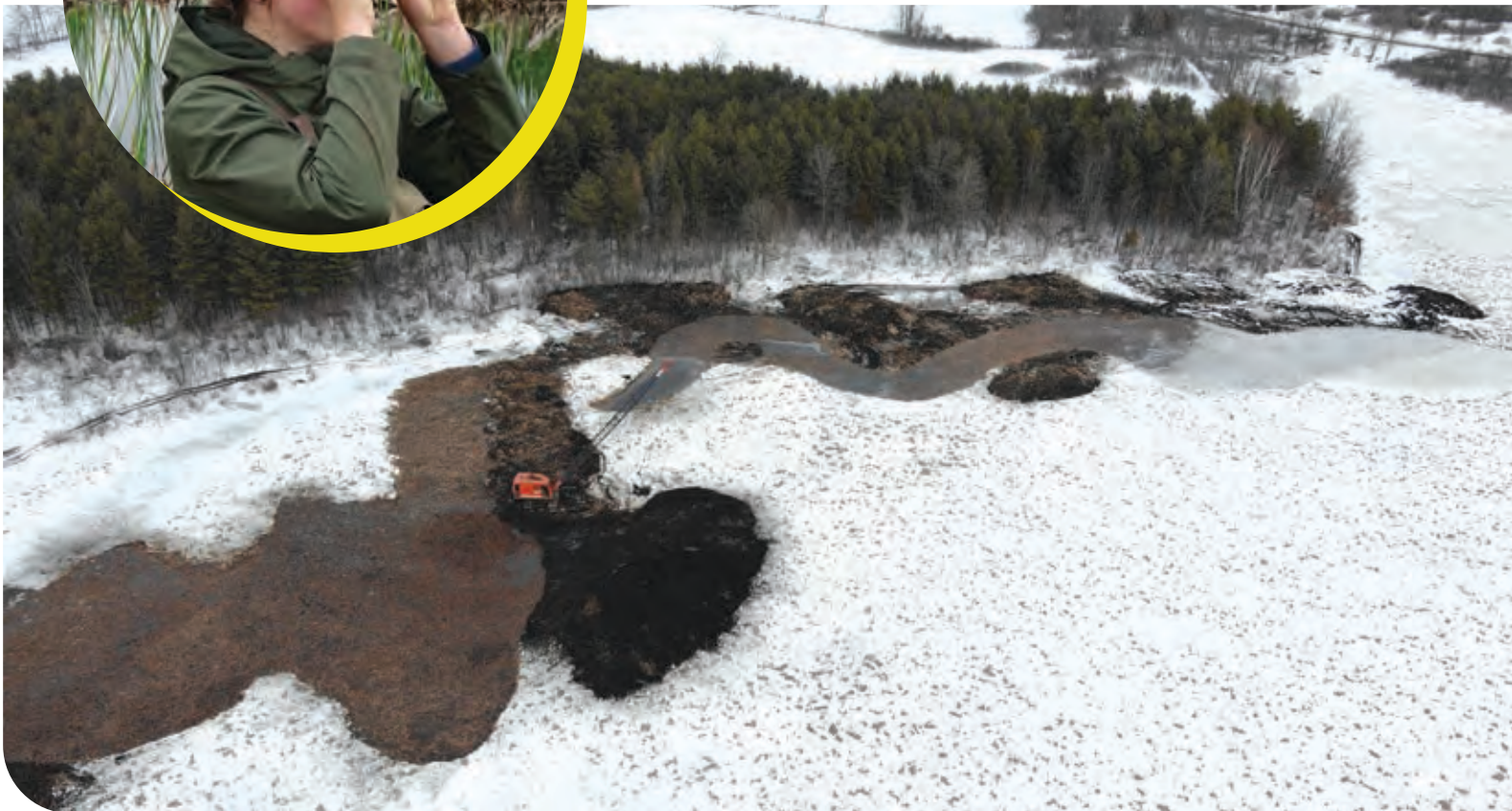
Workers clear open channels and ponds in Hutton Marsh as part of the Motts Mills Wetland Restoration Project in February.
