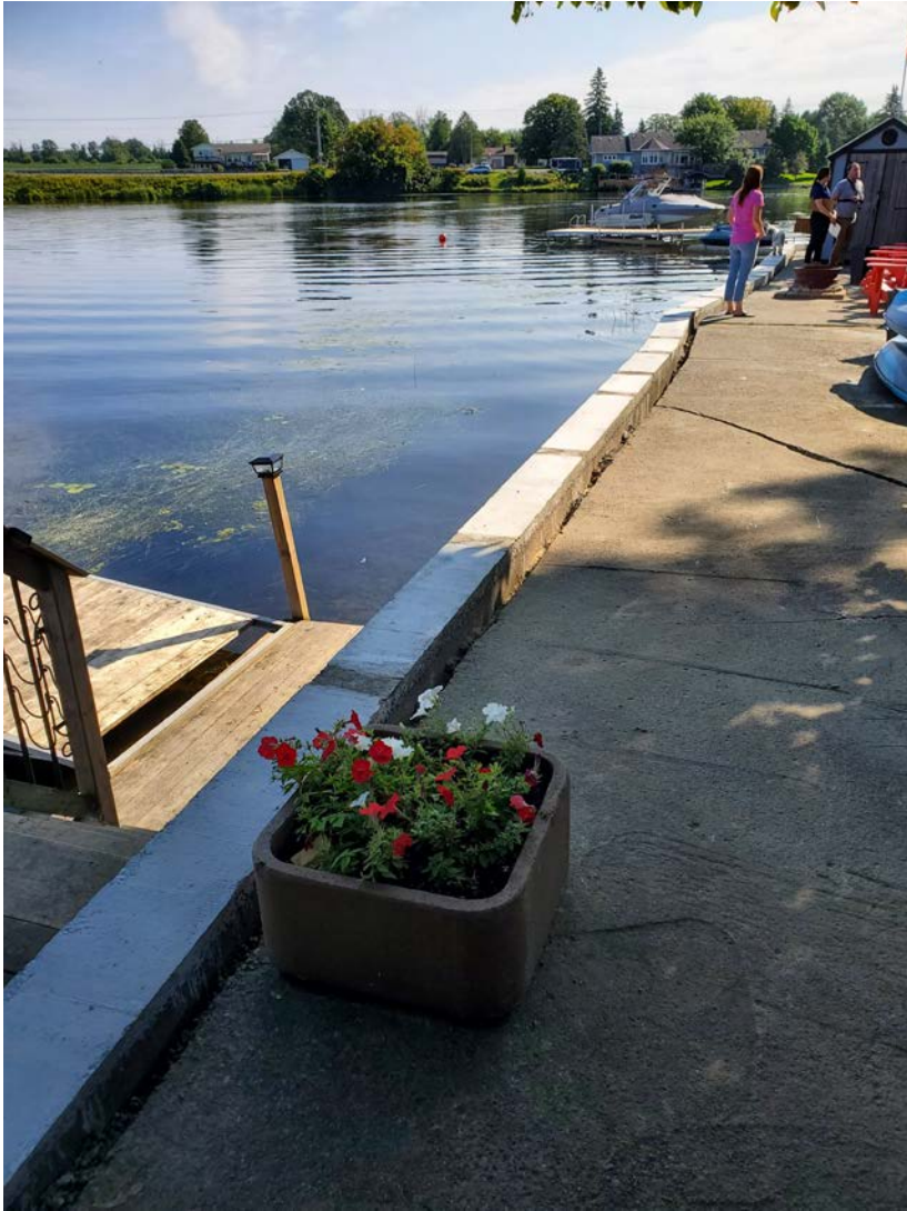
Raised Concrete Sill
