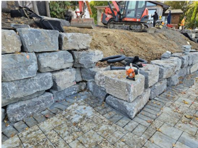
Figure 3. Armor stone retaining wall placed.
