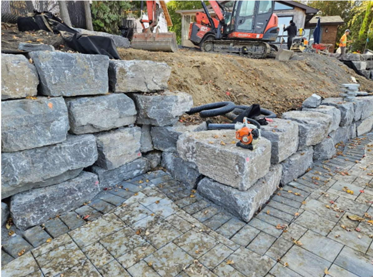
Figure 3. Armor stone retaining wall placed.
