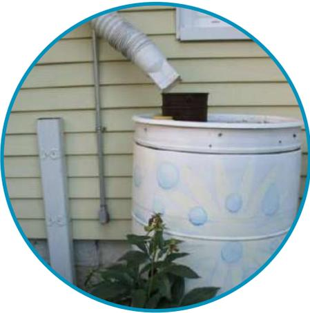
Rain barrels collect rain water directly from downspouts during storm events. This water can be used on gardens, outdoor cleaning or to water the grass, especially during dry periods.
