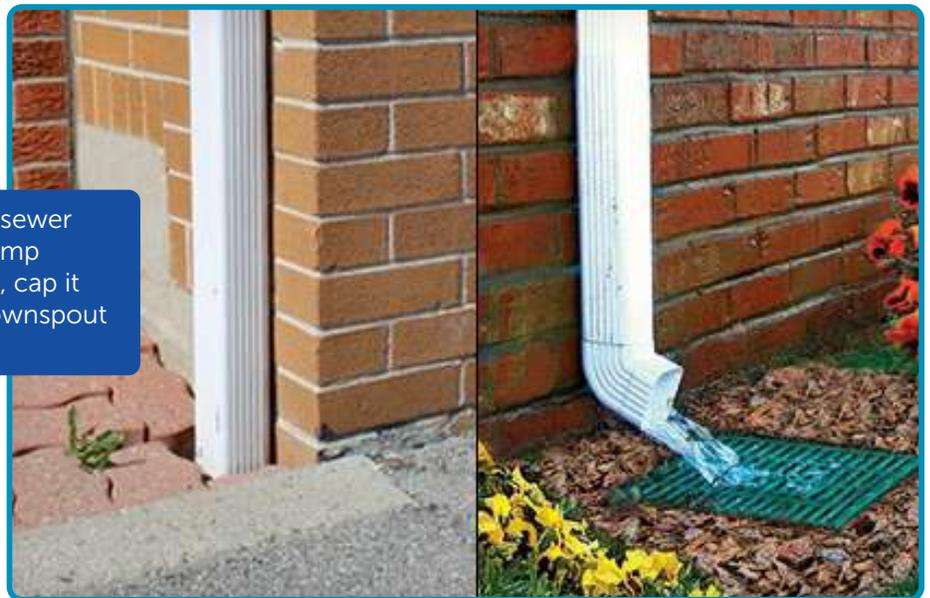
Downspout disconnection and redirection **SLOWS** storm water down, **STORES** rainwater in permeable areas and natural systems, and allows pollutants and sediments picked up by rainwater to be **SOAKED** into the local environment, preventing them from entering local waterways.
