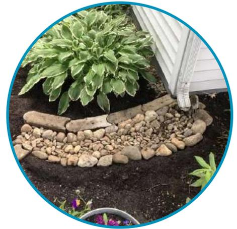
A downspout extender could be directed to an infiltration pit or splash pad to slow water down as it exits the pipe. This reduces erosion of surrounding soils and helps water enter nearby natural systems at a slower rate.
