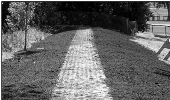
After — upgraded berm with permeable walkway.
