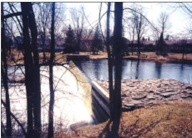
Haggart Island Dam
