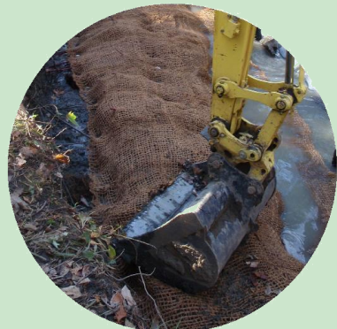
Coir fabric installation
