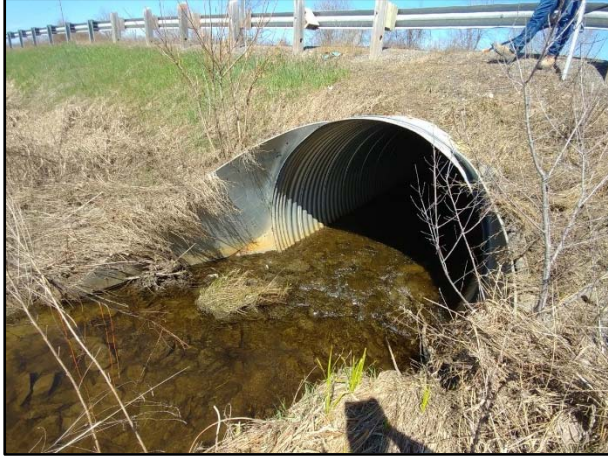
Rideau Road (West of Downey Road) (Upstream)
