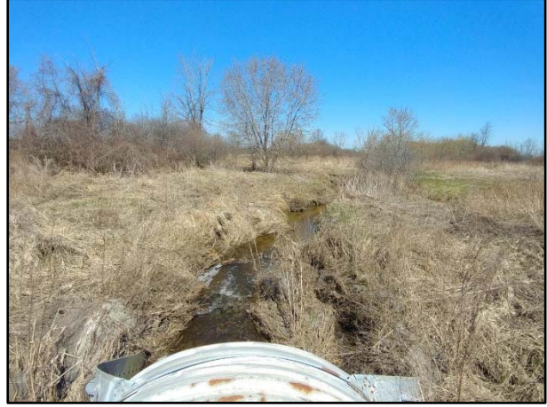
Rideau Road (West of Downey Road) (Downstream)
