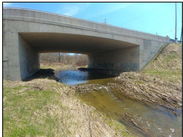
Limebank Road (Downstream)
