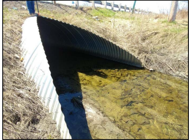
Rideau Road (East of Downey Road) (Downstream)
