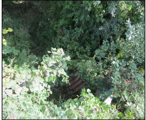
Ashton Station on Kings Tributary (Downstream)
