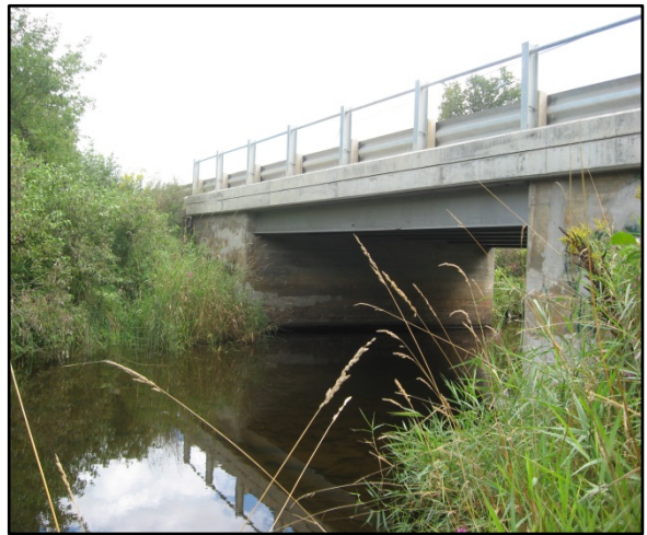
Ashton Station Road (Downstream)
