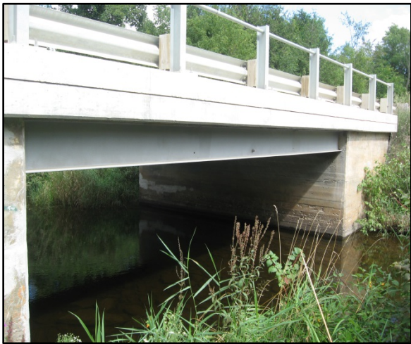
Ashton Station Road (Upstream)
