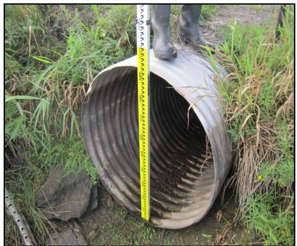
Montigue Boundary road (Downstream)
