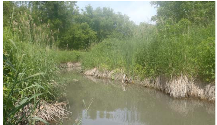
Low level bank undercutting along Black Rapids Creek
