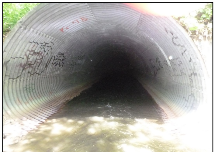
Channelized section of Sawmill Creek under Walkley Road.
