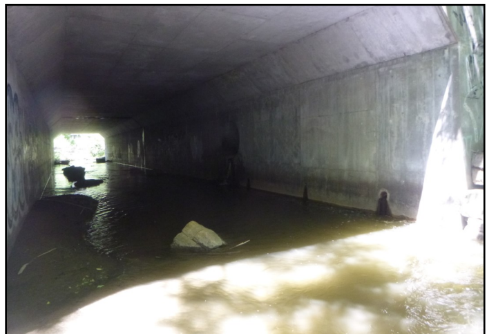
Roadway infrastructure on the transitway along Sawmill Creek.
