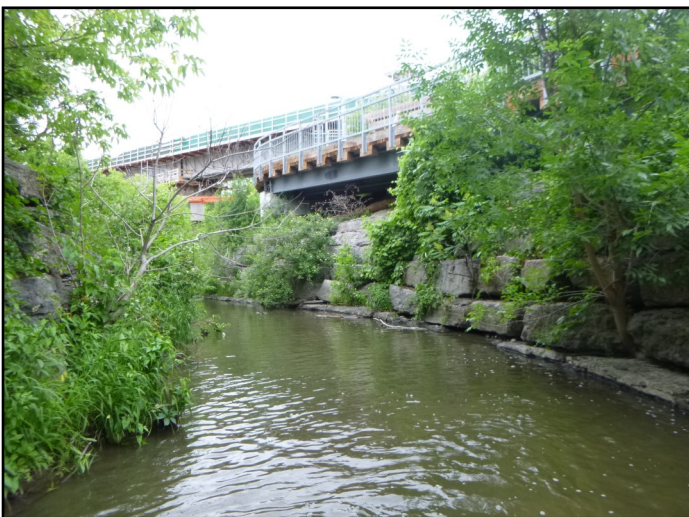
Section along Sawmill Creek with mix land uses including natural forest, scrubland, meadow and urban infrastructure.
