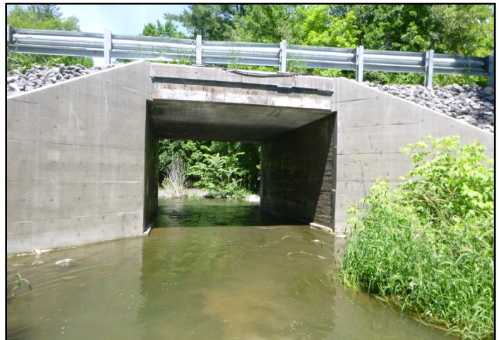
Roadway infrastructure on Watters Road along Cardinal Creek.
