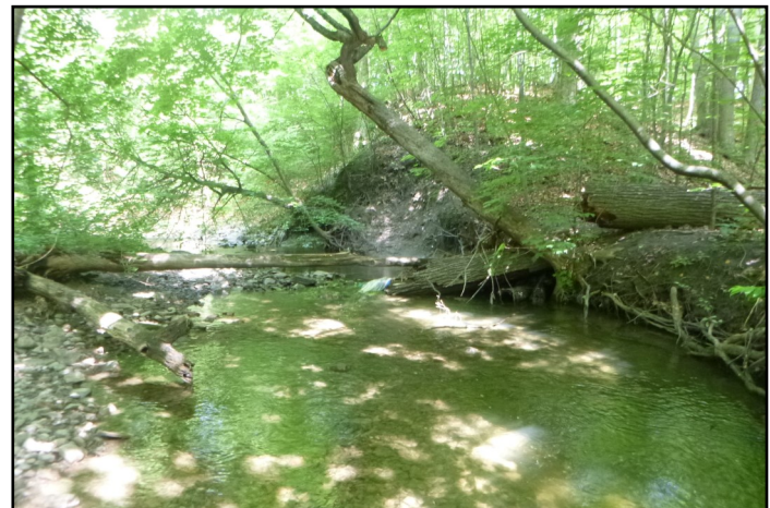
Undercut banks west of Prince of Wales Drive along Barrhaven Creek.
