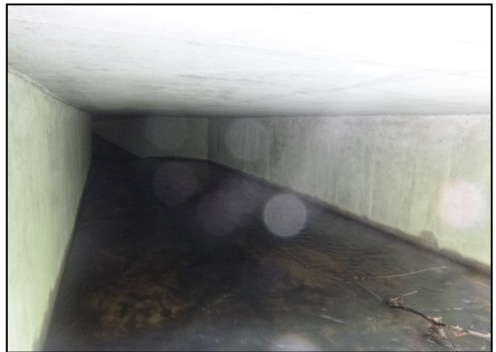
Channelized section of Barrhaven Creek under Prince of Wales Drive.
