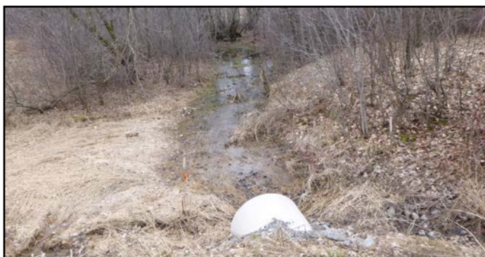
Meadow feature vegetation in a headwater drainage feature on Anderson Road
