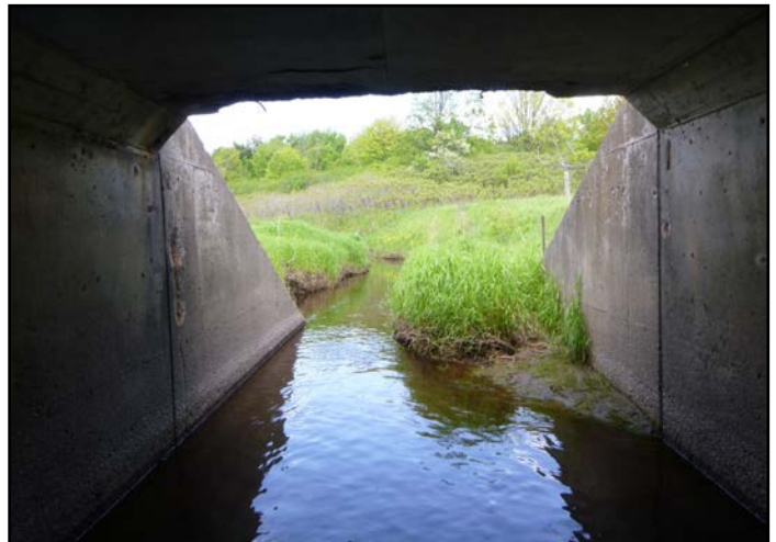
Roadway infrastructure on Walkley Road along Borthwick Creek
