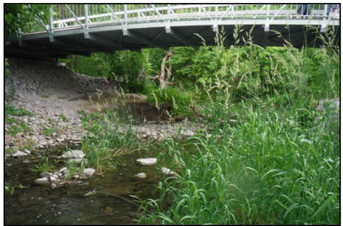
Pedestrian pathway altering a section of Nepean Creek
