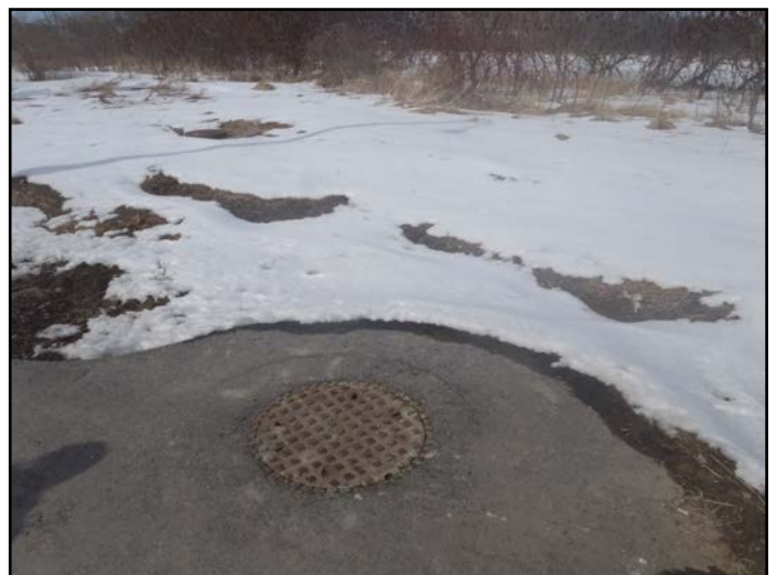
Both top and bottom images show the conditions of the features sampled in 2018. These features are located along Colonnade Road. Once natural features, they are now a part of the stormwater system for Nepean Creek
