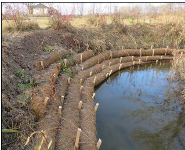
Coir logs were installed (top left) and the protected bank (bottom left) was stabilized with large caliper trees (top right, bottom right)
