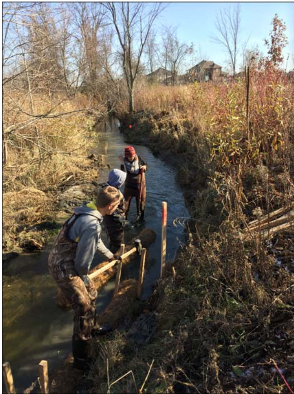
Coir logs were installed (top left) and the protected bank (bottom left) was stabilized with large caliper trees (top right, bottom right)
