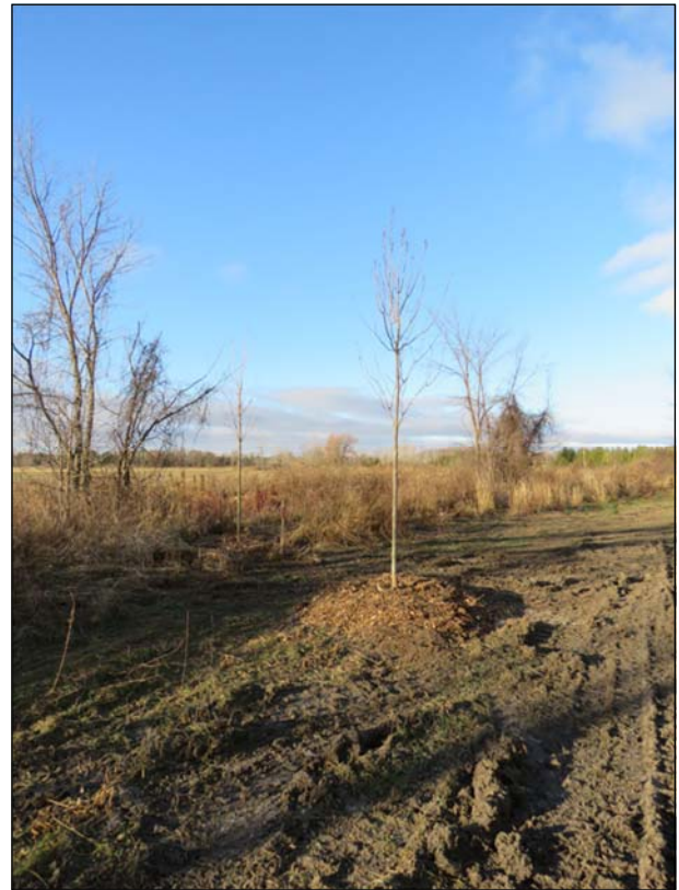
Coir logs were installed (top left) and the protected bank (bottom left) was stabilized with large caliper trees (top right, bottom right)
