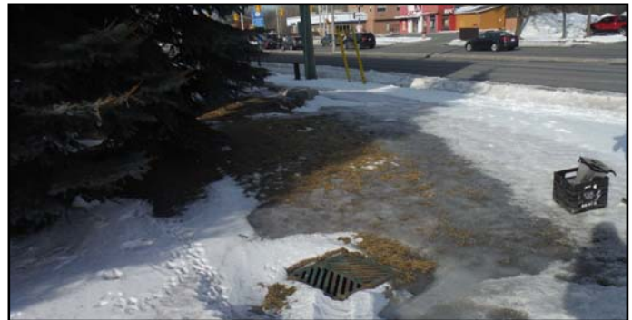
Headwater drainage feature in Pinecrest Creek catchment heavily modified into a stormwater drain along Baseline Road
