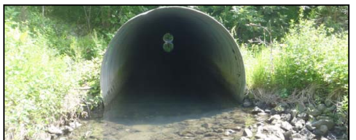
A highly altered stream section flowing through a culvert underneath Woodroffe Avenue
