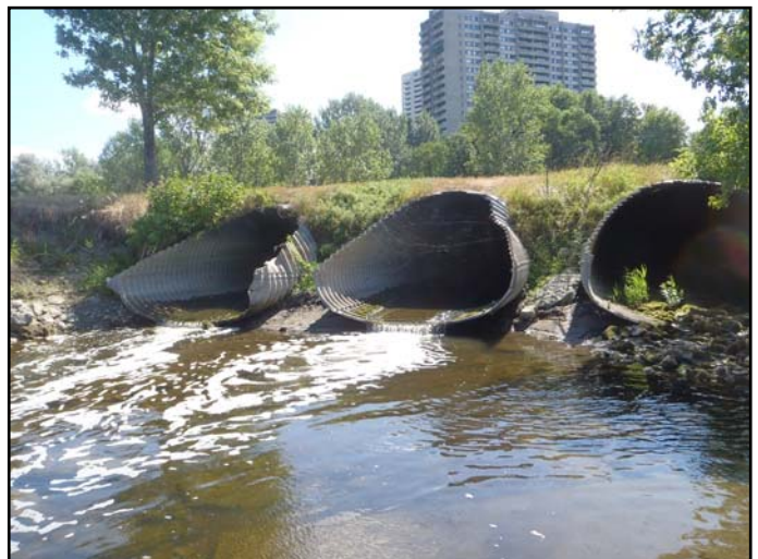
Perched culverts near the Sir John A. Macdonald Parkway (downstream of the Carling Avenue entombment)
