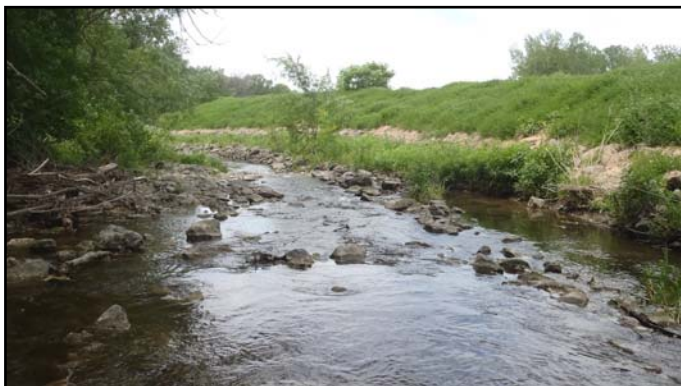
Shoreline re-grading by NCC for erosion control along Pinecrest Creek
