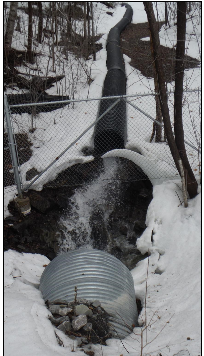
A piped pond outlet headwater drainage feature in the Greens Creek catchment located in the city's east end
