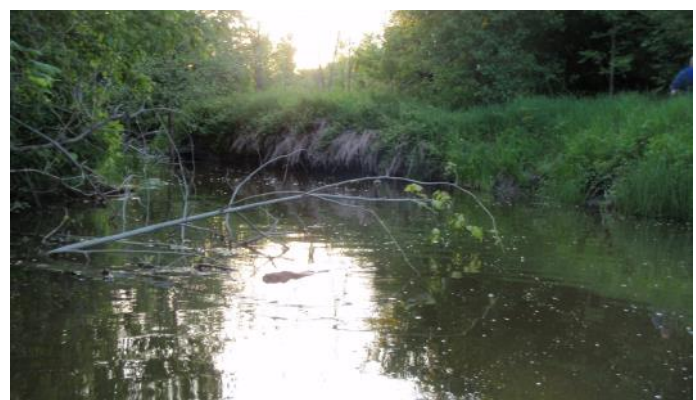
Bank undercutting along Mosquito Creek
