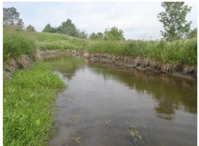
A section upstream of Earl Armstrong Road where a fish habitat enhancement opportunity was identified
