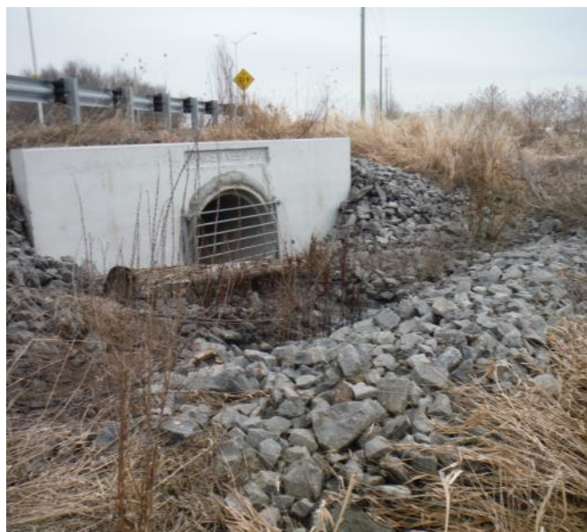
Culvert along Earl Armstrong Road creating a grade barrier
