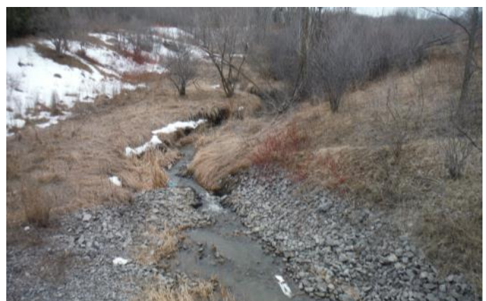
Channel hardening at an HDF site along Limebank Road
