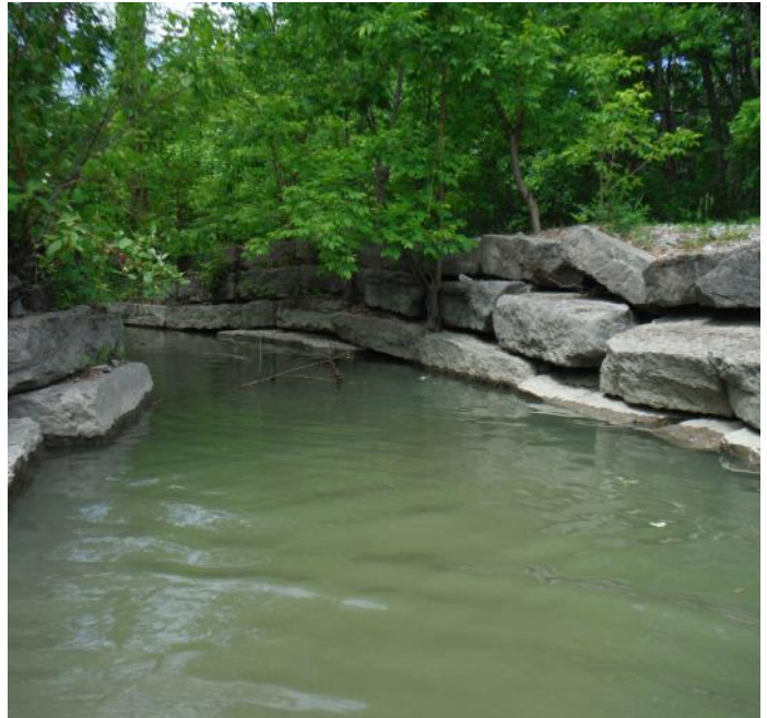
A highly altered section of Bilberry Creek which is channelized and reinforced by armour stone
