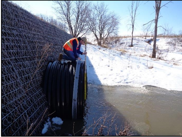
Sarsfield Road near Colonial (Upstream)
