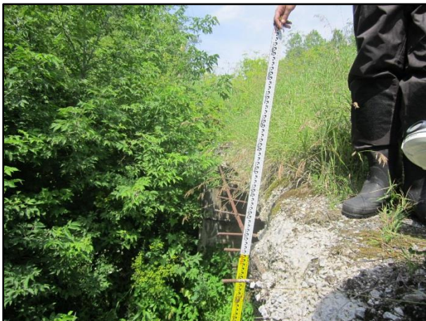
Birchgrove Road south of Étienne (Upstream)
