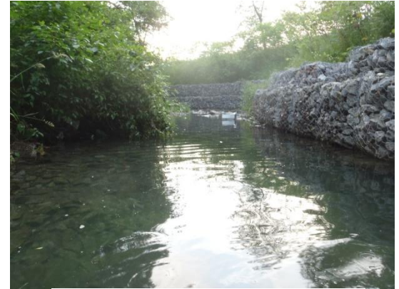
Photo of gabion baskets, a bank alteration
