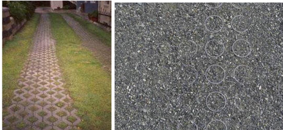
Figure 2: Concrete grid system with grass (left) and plastic grid system with aggregate (right) (CVC & TRCA, 2010)
