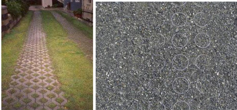
Figure 9: Concrete grid system with grass (left) and plastic grid system with aggregate (right) (CVC & TRCA, 2010)
