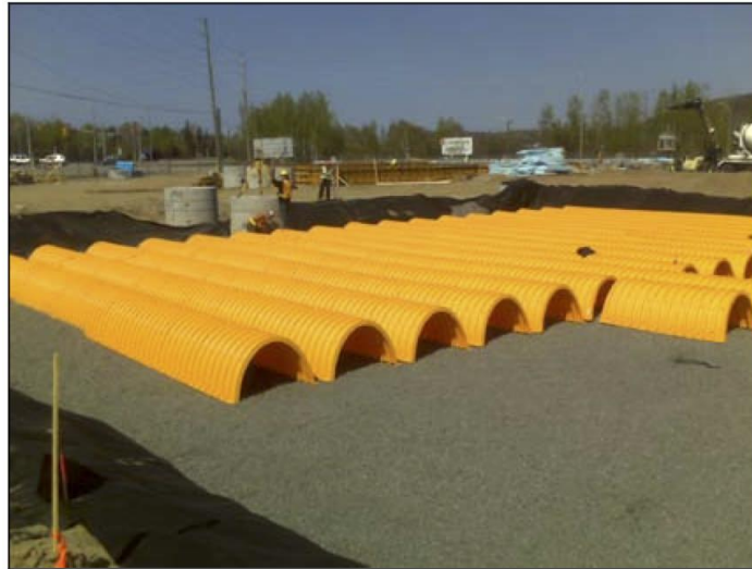
Figure 17: Infiltration chamber example by StormTech (CVC & TRCA, 2010)
