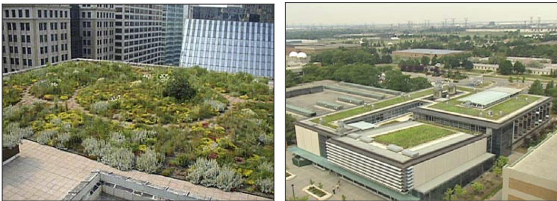
Figure 13: Chicago City Hall Intensive Green roof (left) and York University Extensive Green Roof (right) (CVC & TRCA, 2010)
