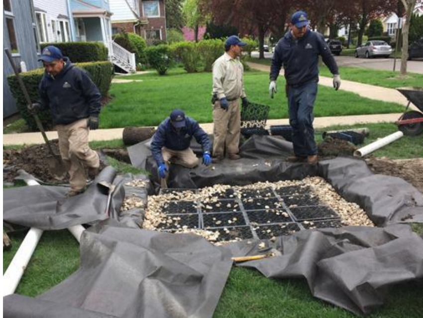
Figure 15: Residential soakaway pit (City of Ottawa, 2022)
