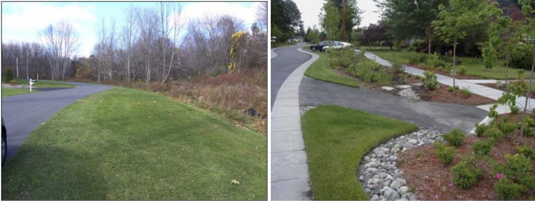
Figure 6: Filter strip along a residential road (left) and as a pre-treatment to a bioswale (right) (CVC & TRCA, 2010)
