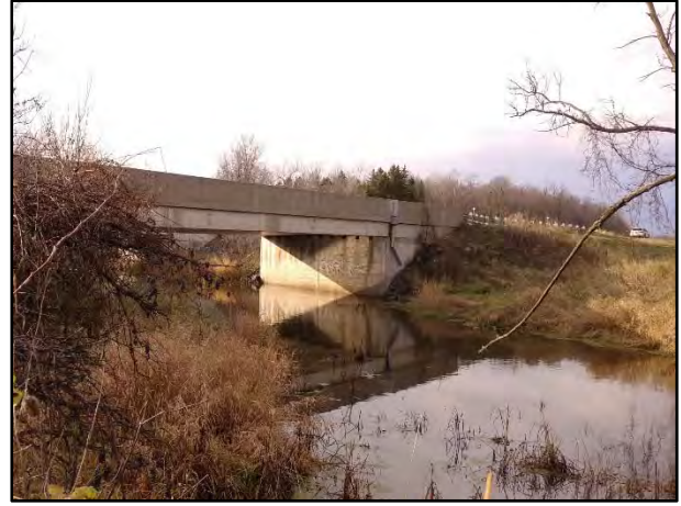
HWY 416 Southbound (Downstream)
