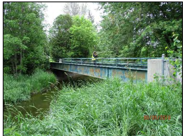
Edward Kidd Park Ped Bridge (Downstream)
