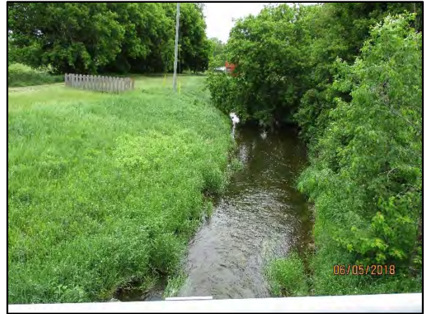
4 th Line Road near Shellstar Drive (Downstream)
