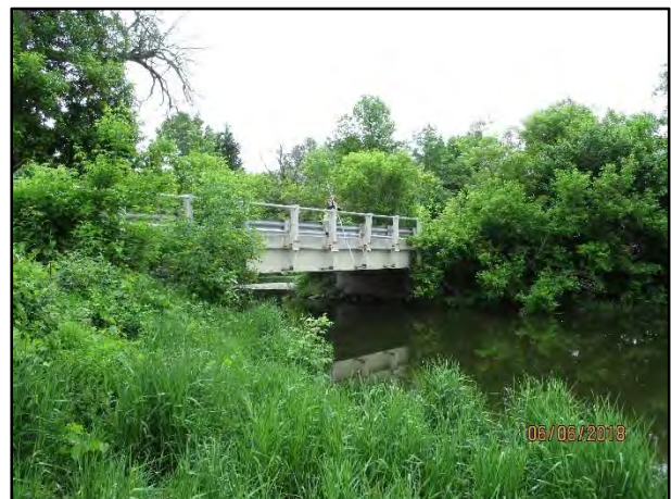
2 nd Line Road South (Downstream)
