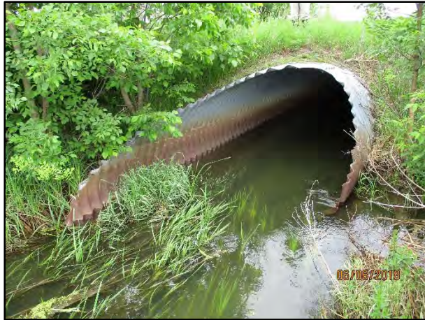
2 nd Line Road South at Roger Stevens (Upstream)
