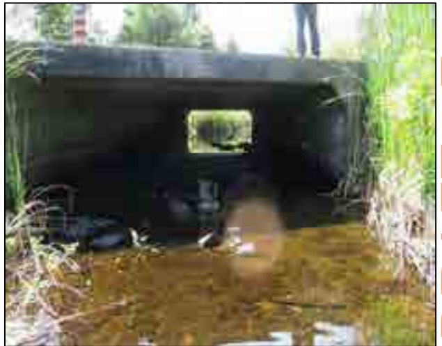
Richmond Rd Culvert (Downstream)
