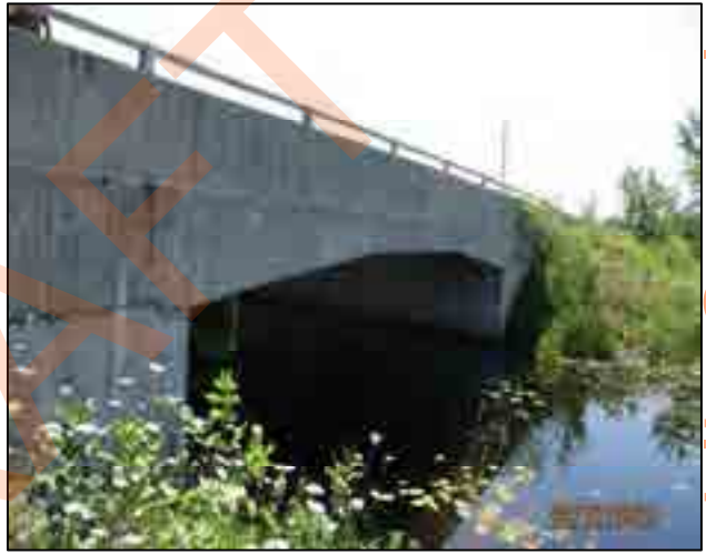
Beckwith 9 Line Bridge (Downstream)
