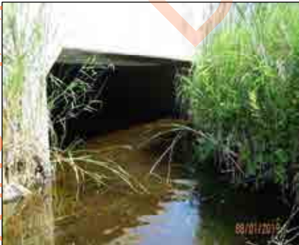
Richmond Rd Culvert (Upstream)
