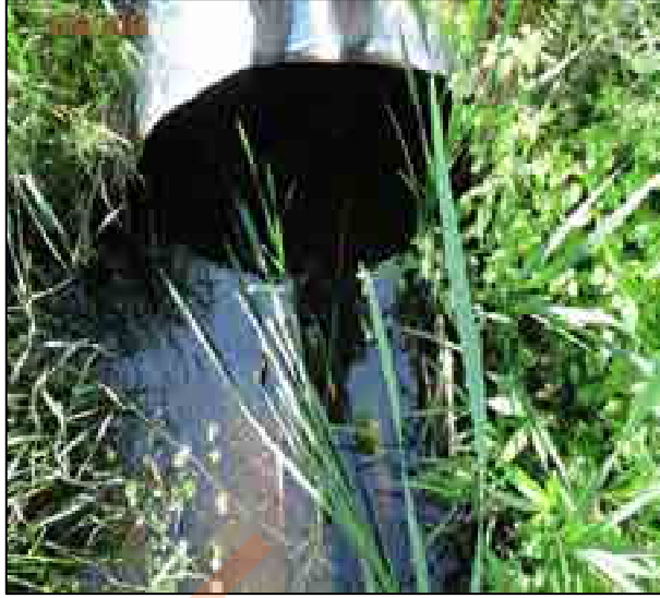
Franktown Swamp Culvert (Downstream)
