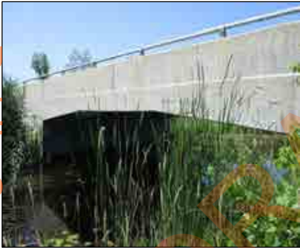
Beckwith 9 Line Bridge (Upstream)
