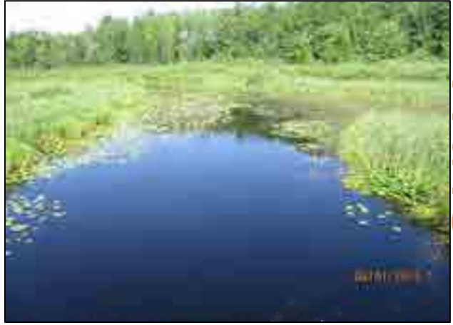
Cemetery Side Road Bridge (Downstream)
