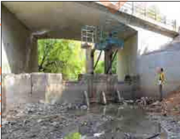
Ashton Station Dam (Upstream)
