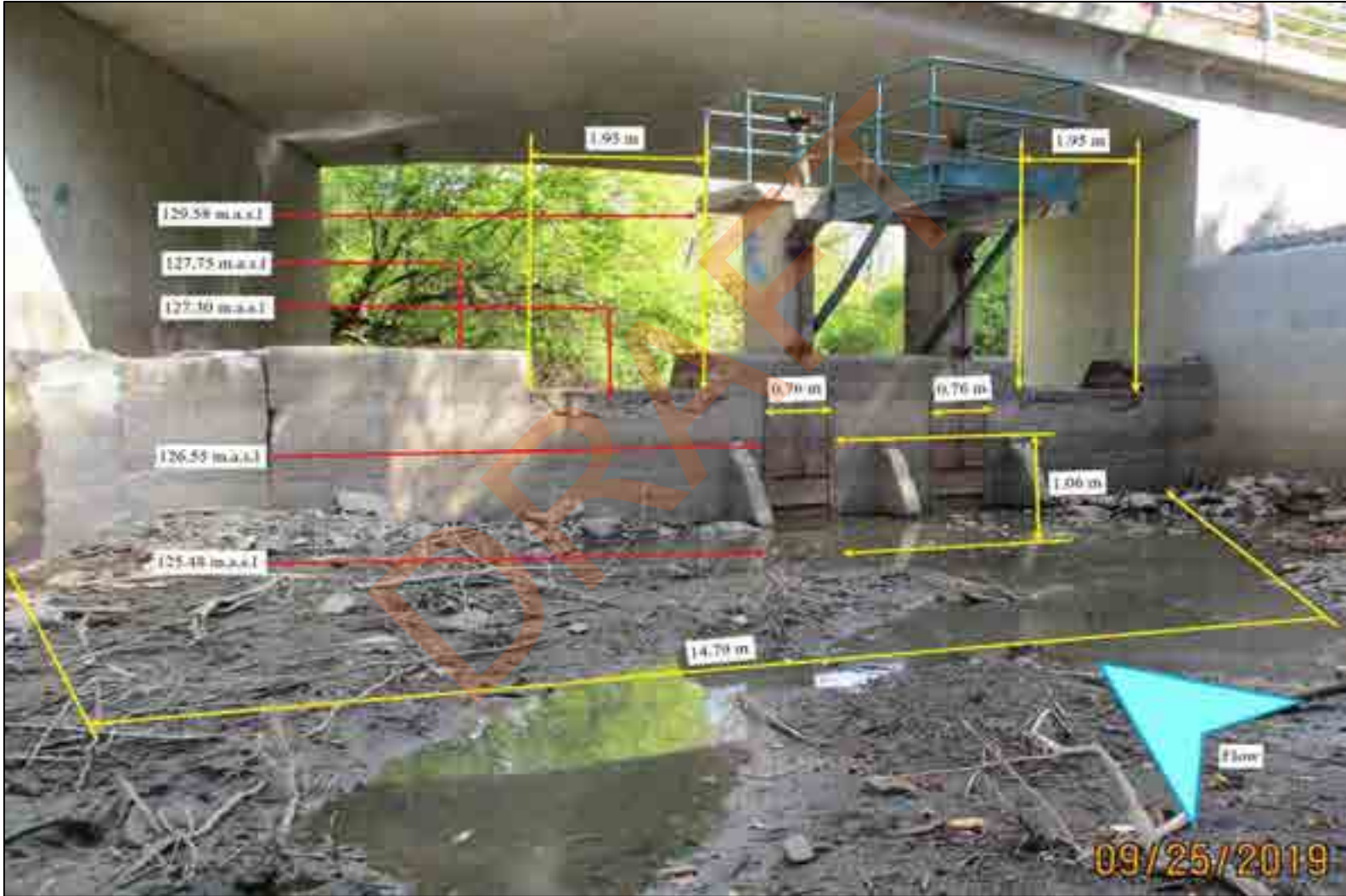
Figure 20 Ashton Station Dam
