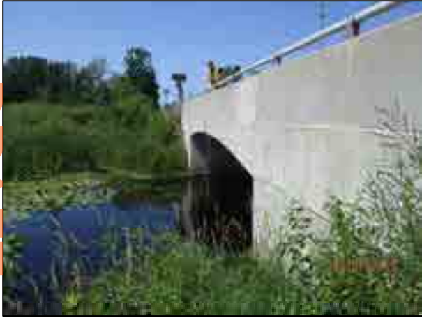
Cemetery Side Road Bridge (Upstream)
