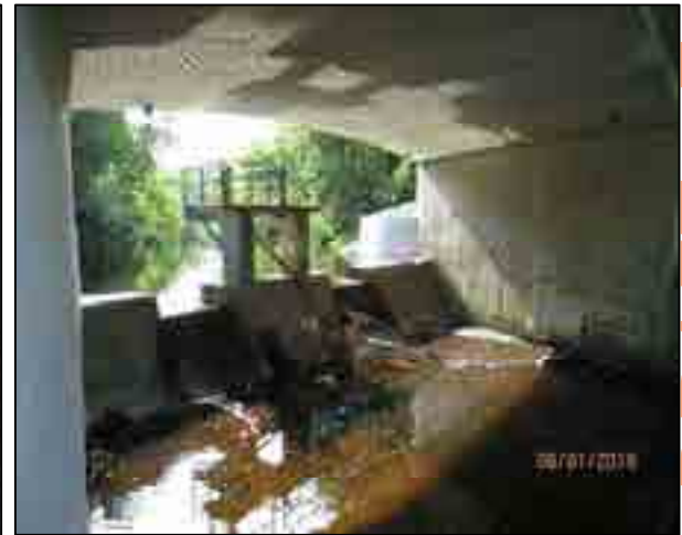
Ashton Station Dam (Downstream)
